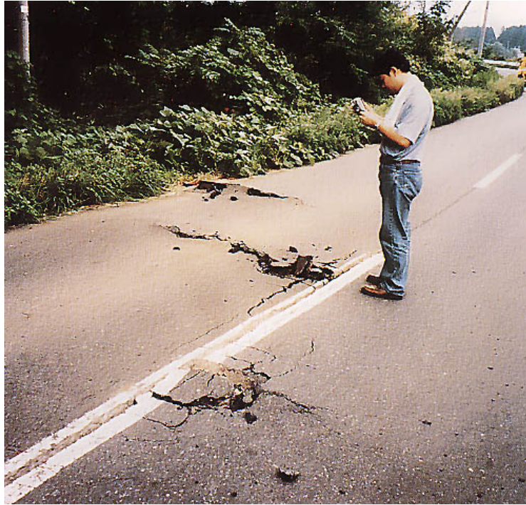
Photo 3 Buckled pavement
