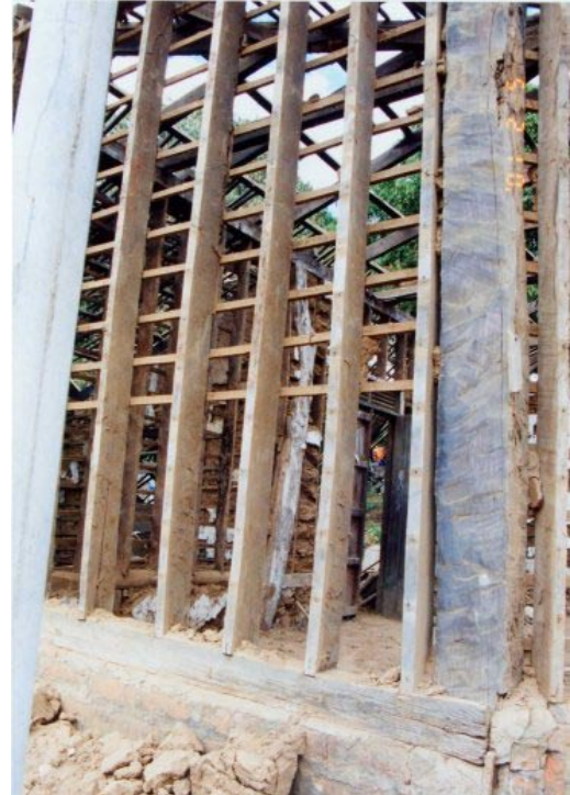
Figure 3.12. Bahareque structure that suffer mud spalling.
