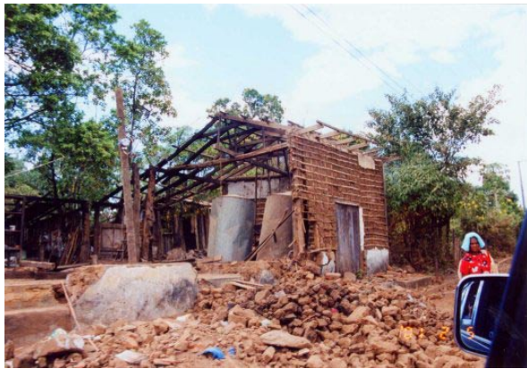
Figure 3.19. Collapsed bahareque house.
