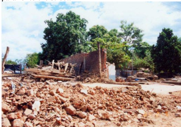
Figure 3.15. Completely collapsed adobe house.
