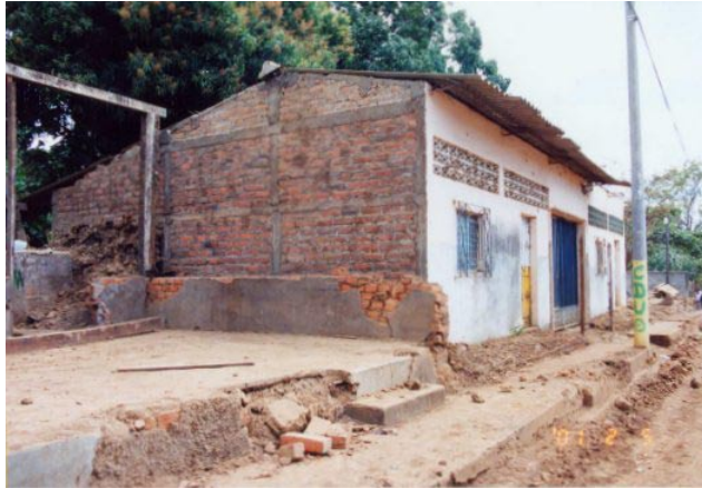
Figure 3.17. Adobe house completely flattened next to a reinforced masonry structure that did not suffer any damage.
