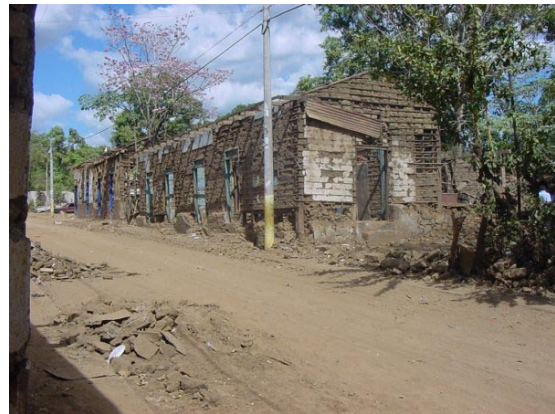
Figure 3.26. Bahareque structure damaged by the earthquake.
