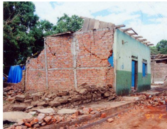
Figure 3.16. Collapsed reinforced masonry wall. The separation of the walls from the transverse walls can be observed in the two buildings shown in the photograph. The street direction is approximately NE-SW.
