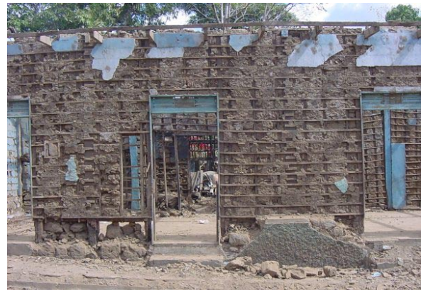
Figure 3.27. Details of the walls of the house in Figure 3.26 . Notice the poor foundation detail.
