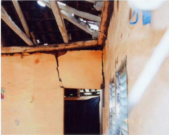
Figure 3.23. Interior of the building shown in Figure 3.21 . Vertical cracking of spandrels over the door head can be observed.
