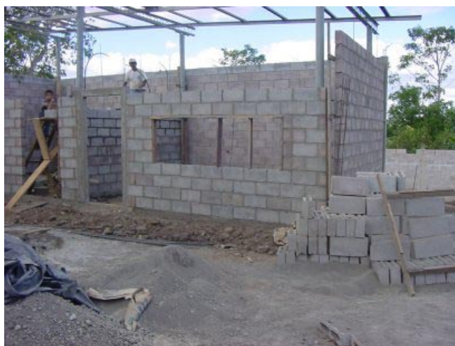
Figure 3.1. Reinforced masonry house with concrete blocks
