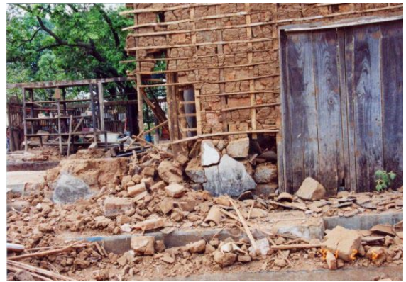
Figure 3.20. Detail of the poor foundation of house in Figure 3.19 .
