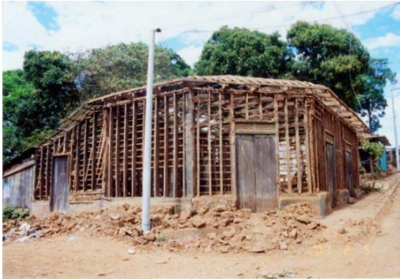
Figure 3.12. Bahareque structure that suffer mud spalling.
