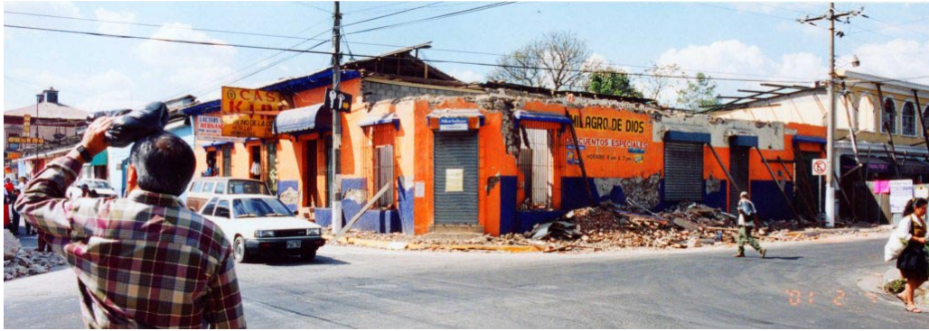
Figure 3.47. Adobe construction suffered damage at Nueva San Salvador.
