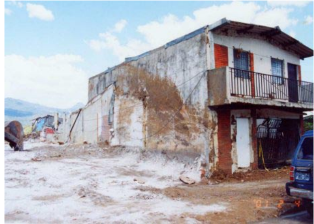
Figure 3.44. Dwelling on the border of the landslide. Neither the earthquake ground shake nor the landslide affected this dwelling.
