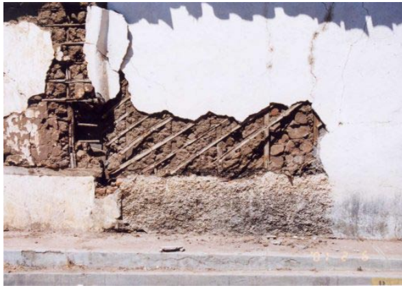
Figure 3.37. Spalling of the mud cover in a bahareque dwelling. The wall presents horizontal, vertical, and diagonal canes.
