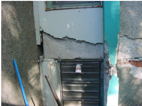
Figure 3.48. Finishing spalling. The seismic joint between two adjacent buildings was 5cm. No evidence of pounding was observed.
