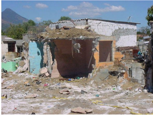
Figure 3.43. Concrete block dwelling affected by the landslide at Las Colinas. There is still soil on top of the roof.
