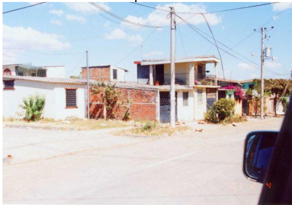
Figure 3.45. Reinforced masonry dwellings few meters away from the landslide did not suffer any damage.
