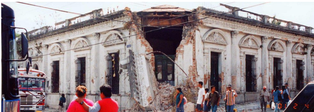
Figure 3.46. Unreinforced masonry structure suffered structural damage at the historical center of Nueva San Salvador.
