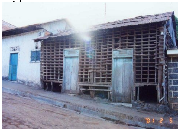
Figure 3.30. Bahareque house that lost all its mud walls.
