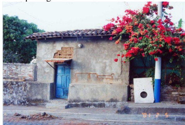
Figure 3.31. Bahareque house exhibiting mud cover spalling and vertical cracking at the connection between two perpendicular walls.
