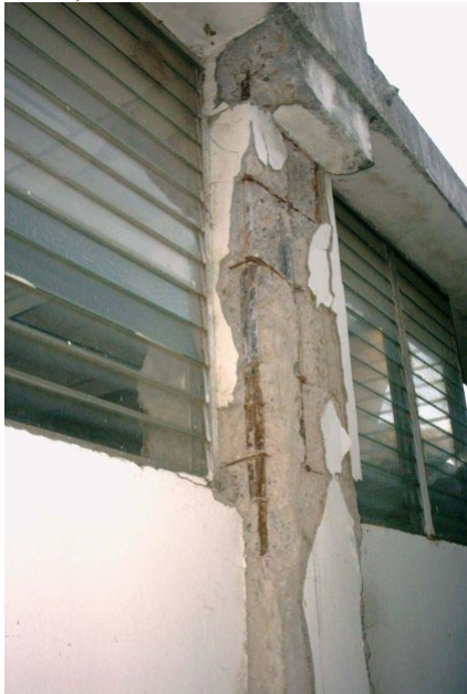
Figure 3.35. Typical damage in the TELECOM building. Thin concrete cover spalled (Courtesy Mr. LaFolie).
