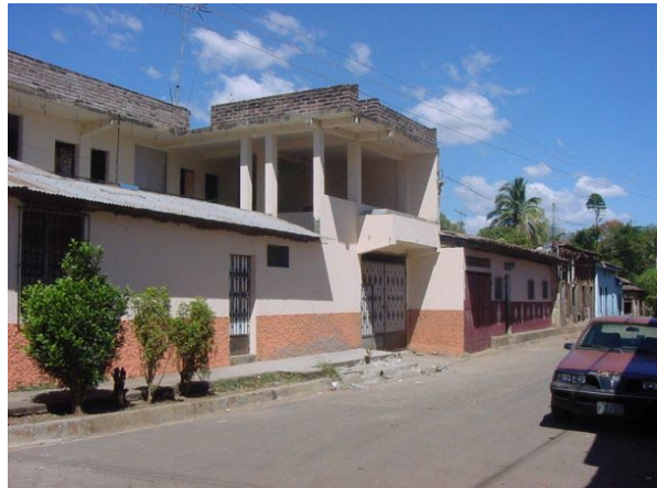
Figure 3.38. Reinforced masonry structure performed well.
