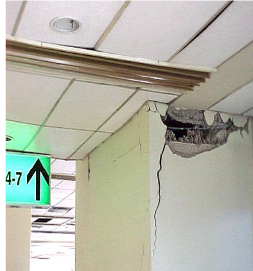
Figure 4.36. Reinforced masonry wall near boarding gates cracked along mortar block joints
