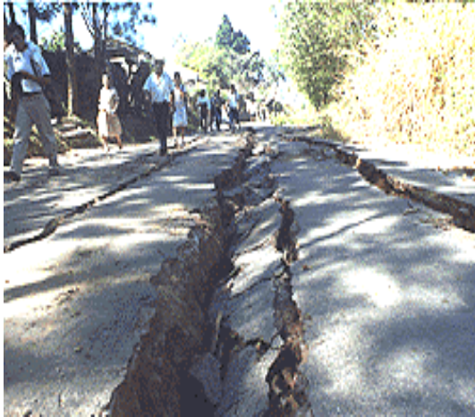
Figure 4.32. Longitudinal cracks in road to Comasagua, La Libertad
