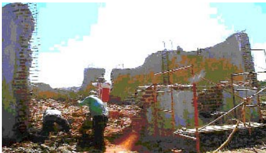
Figure 4.19. Reinforced Masonry wal of “ Las Colinas del Norte ” tank
