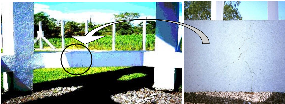
Figure 4.20 Damage to a RC water tank tower (Apopa) Left: Rectangular water tank Right: Cracks on beam column joints
