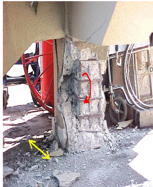
Figure 4.38. Crumbled short RC column
