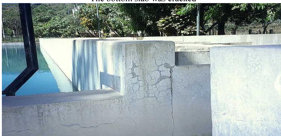
Figure 4.23. Cracks on construction joints on RC walls surrounding filtering facility
