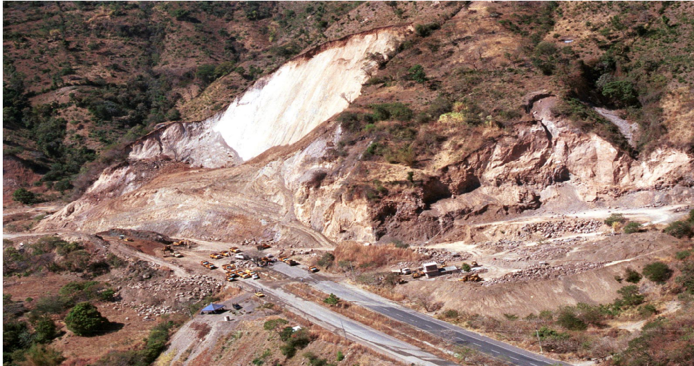
Figure 4.25. Landslide at “Leona” blocking the Pan-American Highway.
