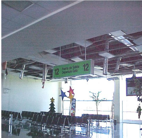
Figure 4.35. Damage to ceiling panels (passengers waiting room)
