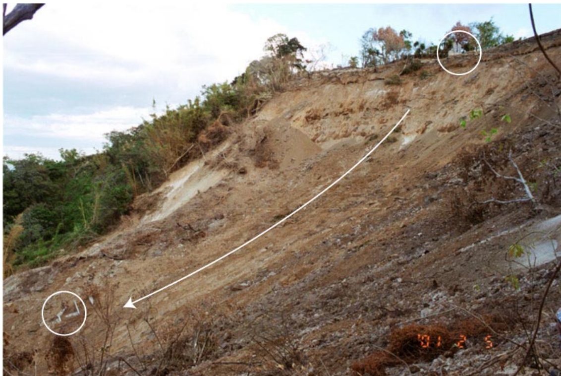
Figure 2.25. Fallen block fence
