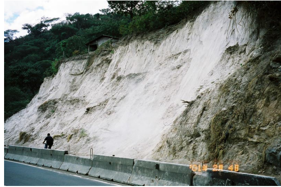
Figure 2.60. Exposed failure surface of pyroclastic flow sediment.
