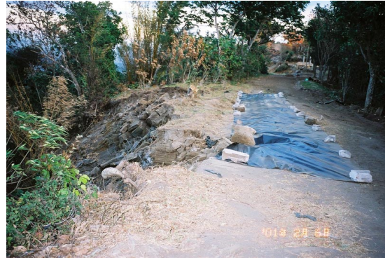
Figure 2.55. Longitudinal crack at Site III
