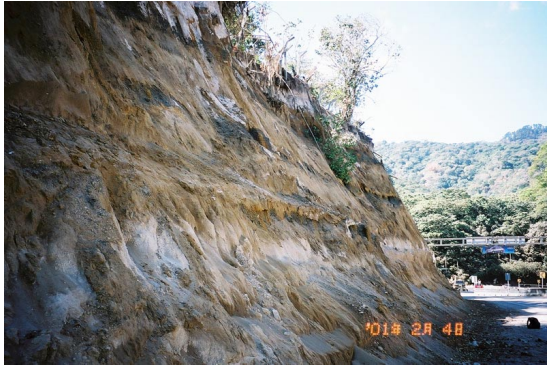
Figure 2.59. Failure surface exhibiting an arrangement of volcanic products in strata. Two lapilli tuff layers (dark gray) lie between the loose pumice soil sediment (ocher).
