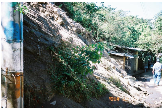
Figure 2.62. Slope failure on weathered tuff
