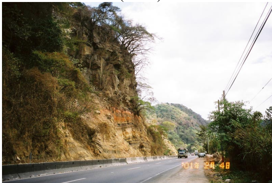
Figure 2.59. Failure surface exhibiting an arrangement of volcanic products in strata. Two lapilli tuff layers (dark gray) lie between the loose pumice soil sediment (ocher).
