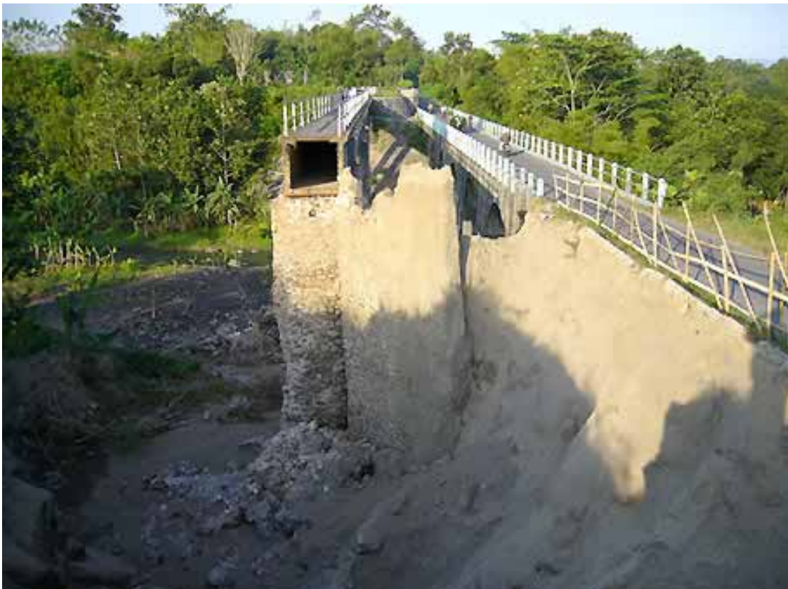
Fig. 3. Mataram canal bridge: Soil mass of right embankment behind masonry abutment has gone.
