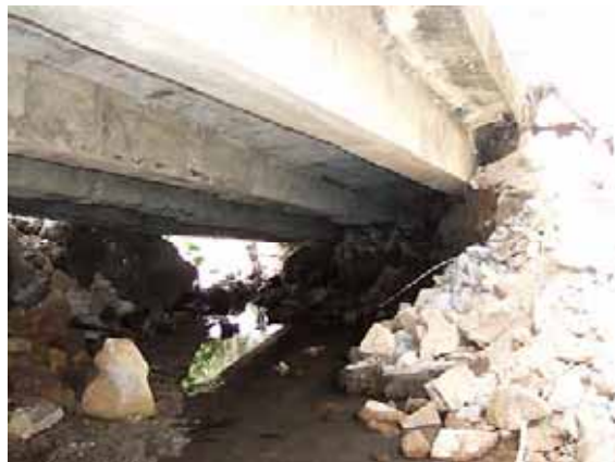
(c) Four simple beams support the deck.
