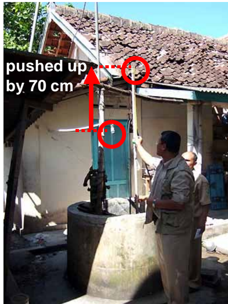
(a) S7deg. 57.416 min, E110deg. 18.291 min plastic pipe was pushed 0.7m up.
