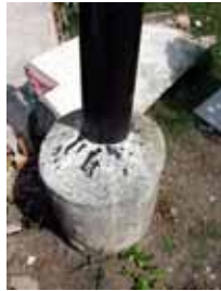
Fig. 1. No clear cracking of lamppost pedestal was found. (Pesu, Klaten)
