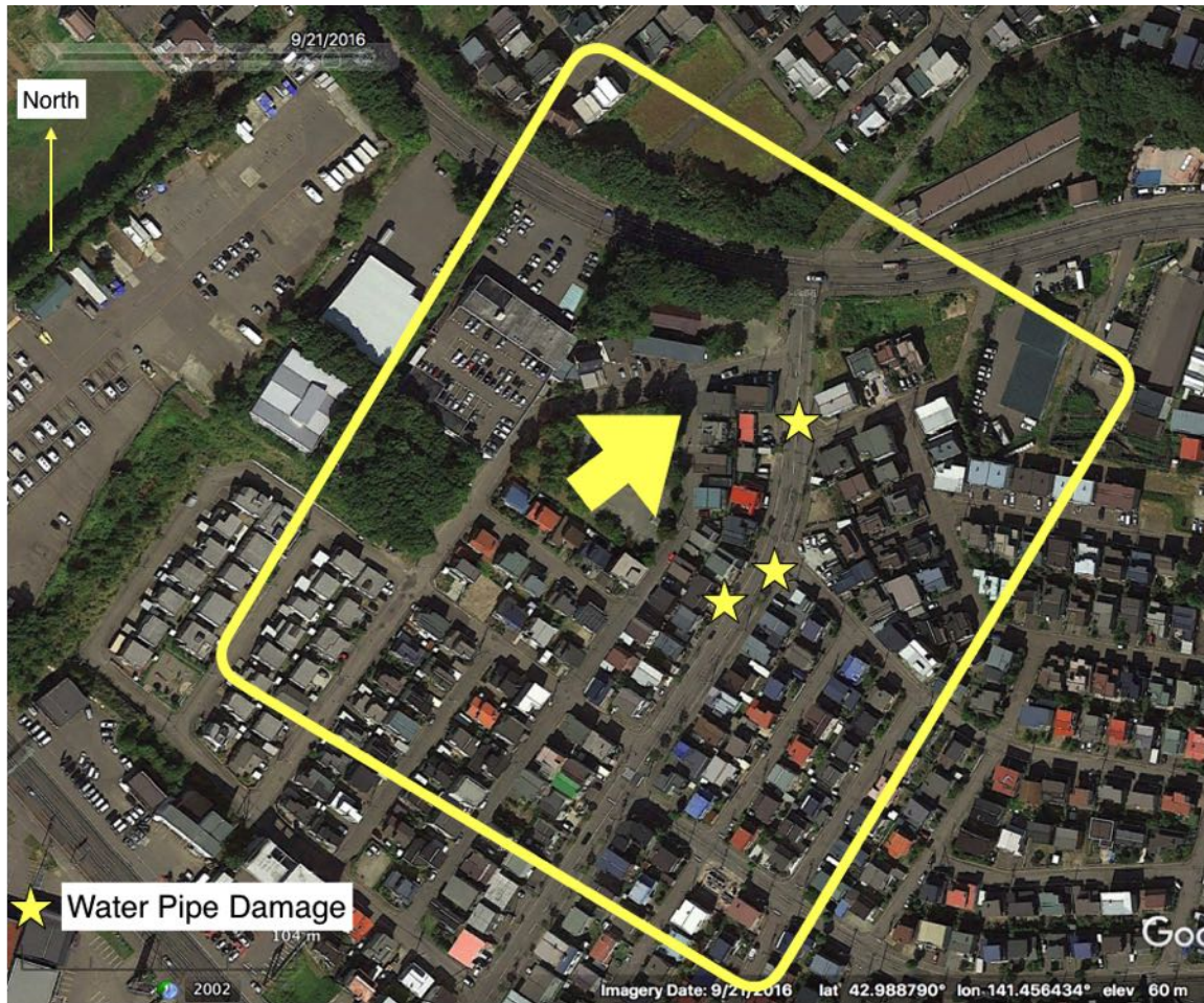
Figure 2-18. Liquefaction zone in Kiyota-Ward (latitude 42.9888 long 141.4564)
