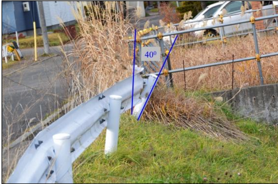
Figure 6-15. The support pole rotated about 40^{\circ} .
