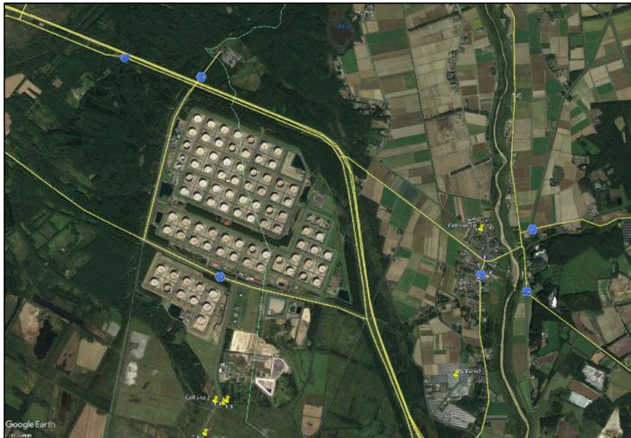
Figure 4-10. Aerial view of the tank farm for oil storage. A total of 82 tanks in this facility. (Source: Google Earth)
