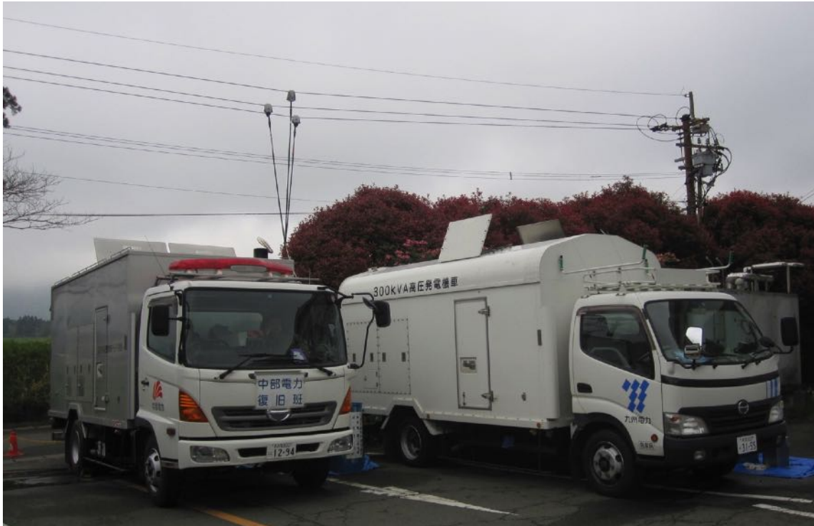
Figure 3-48. Hooking up an Emergency Generator to a Distribution Primary
