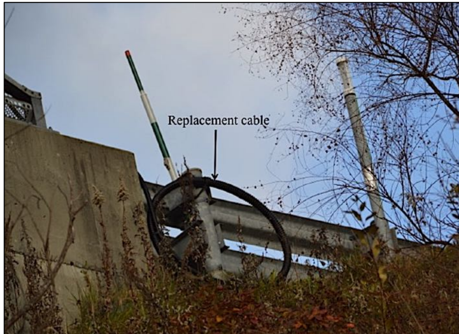
Figure 6-4. Replaced cable temporarily strapped to the guard rail of the expressway
