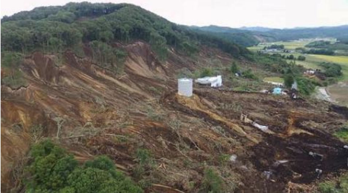
Figure 5-16. Landslide Impact on Atsuma WTP, Oblique View (credit: https://www.jiji.com/jc/article?k=2018091200862&g=wth )
