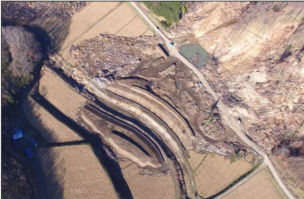
Figure 7-24. This shows the extent of the landslide damage. The road was covered by the creek was also blocked. A retaining wall was temporary built to prevent mud flowing to creek. (Source: Masataka Shiga)
