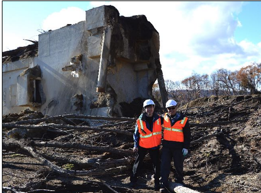
Prof Konagai (Left) and Alex Tang (Right) in front of the destroyed stair column of the Water Treatment Plant (see Chapter 5). The piles were pulled out by the landslide. (Credit: Mr. Ingemansson)
