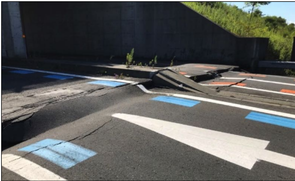
Figure 7-22. Mukawa Interchange road surface just beneath the overpass (Credit: MLIT)
