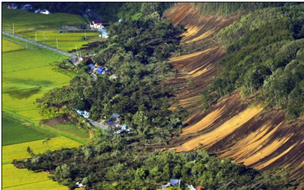
Figure 6-3. The massive landslide destroyed the road and the utility poles for both power and telecom connections. (Credit: Masataka Shiga)
