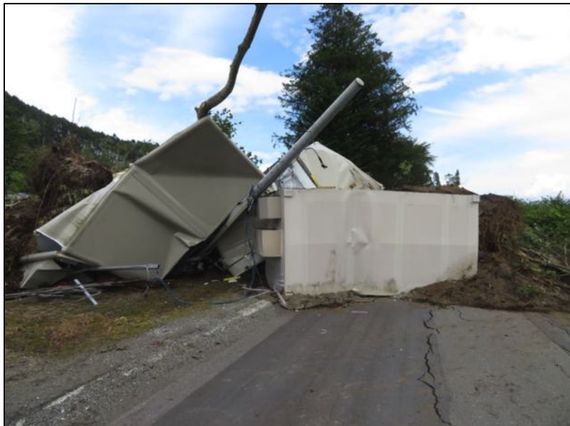
Figure 6-7. Remote Office destroyed by landslide. (Source: Prof Suzuki of Toyo University)
