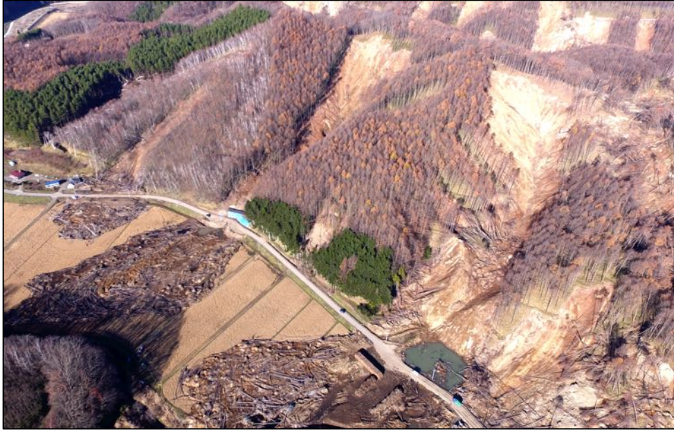
Figure 7-23. Three locations on this secondary road were covered by landslide. The one on the right is the largest. The road surface was not repaved as of mid-November 2018. (Source: Masataka Shiga)
