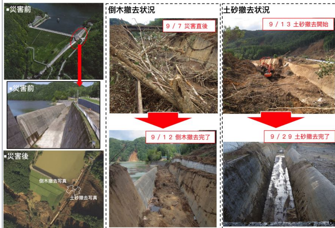
Figure 5-26. Repair of Spillway, Upper Atsuma Reservoir (Credit: MILT)
