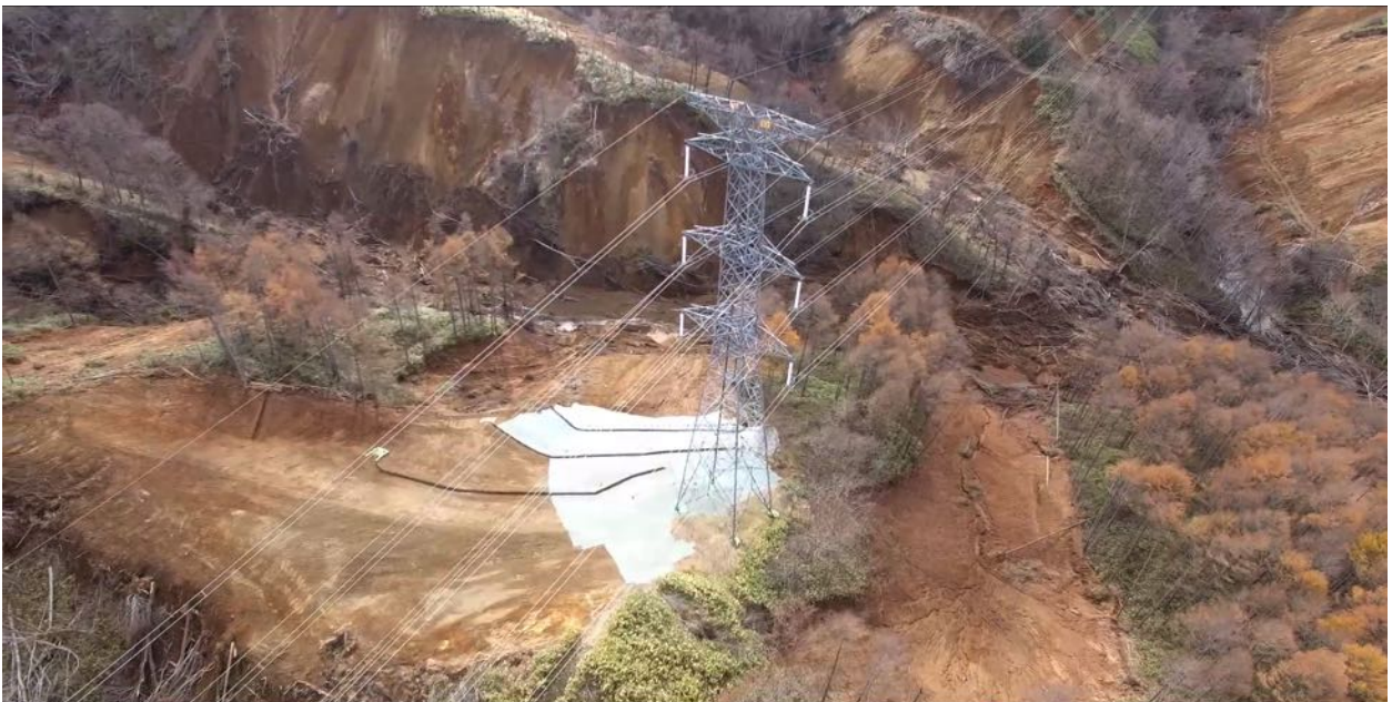
Figure 3-22. Aerial View looking Southeast (credit: Shiga)
