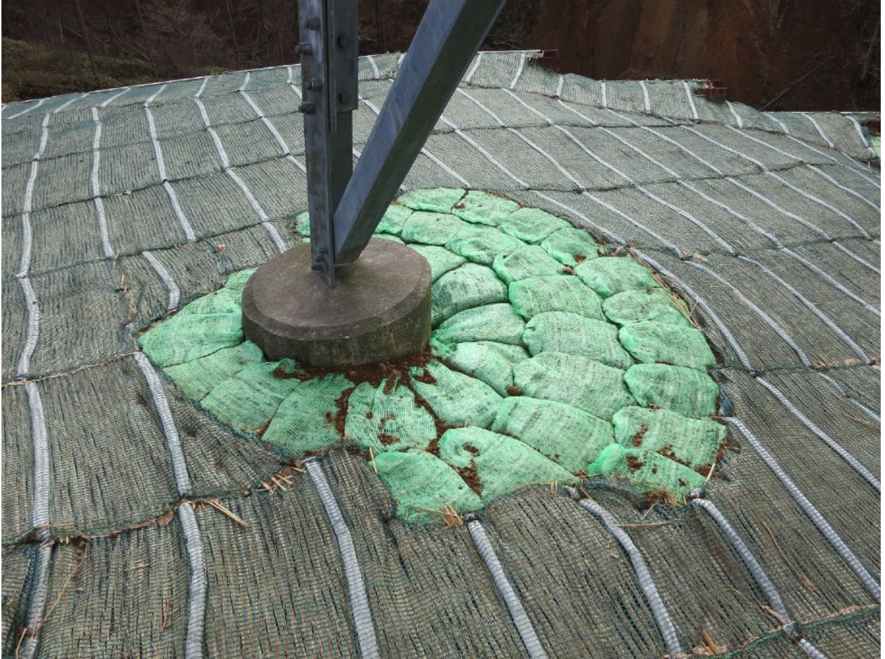
Figure 3-25. Typical Repair at Tower Foundation within Landslide
