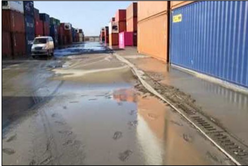
Figure 8-5. Liquefaction at the International Container Port (Source: MLIT)
