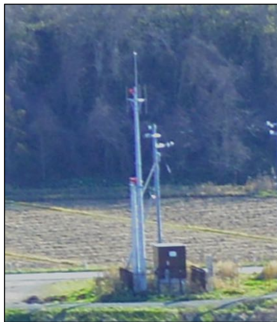
Figure 6-9. View of the cabinet from the ruins of the WTP, note fence was added
