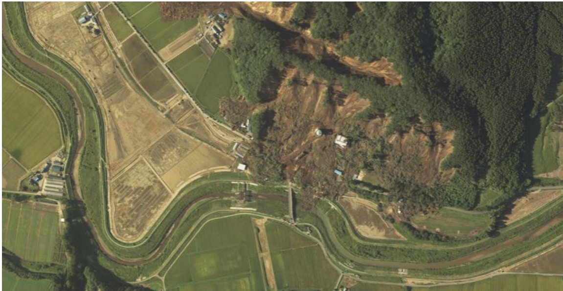
Figure 5-15. Landslide Impact on Atsuma WTP (credit: Google)
