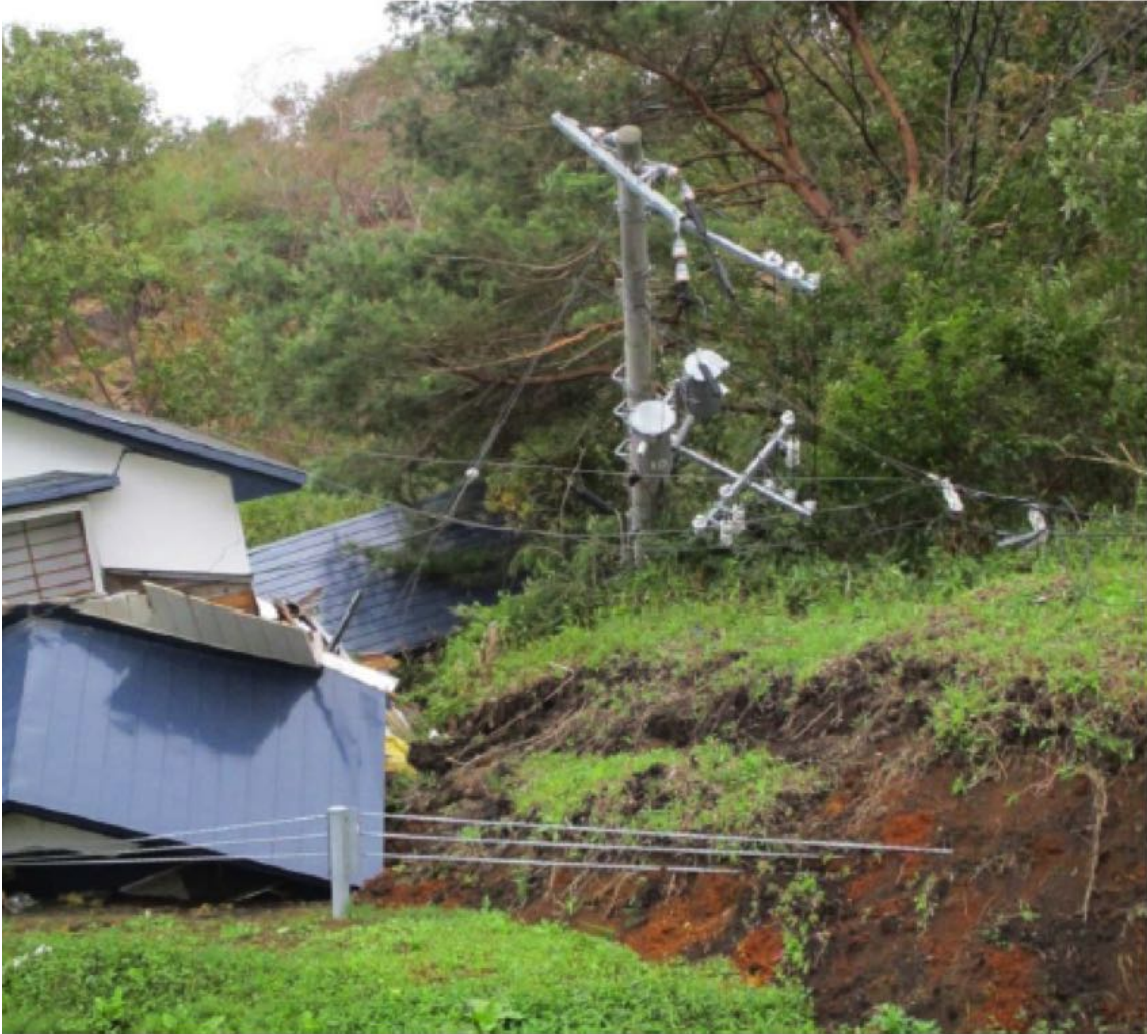
Figure 3-45. Toppled Distribution Pole due to PGDs (Atsuma-Cho) (Credit: HEPCO)
