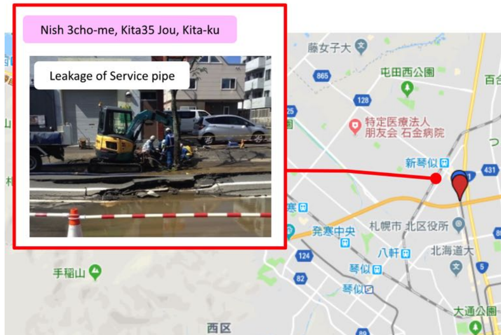
Figure 5-13. Service Line Repair, North of JR Sapporo Station (credit: Kubota)
