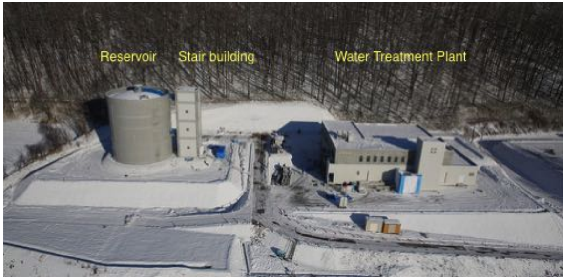
Figure 5-14. Atsuma New Water Treatment Plant (Tomisato) (photo credit: http://www.maruhiro-nozawagumi.com/sekou.html )
