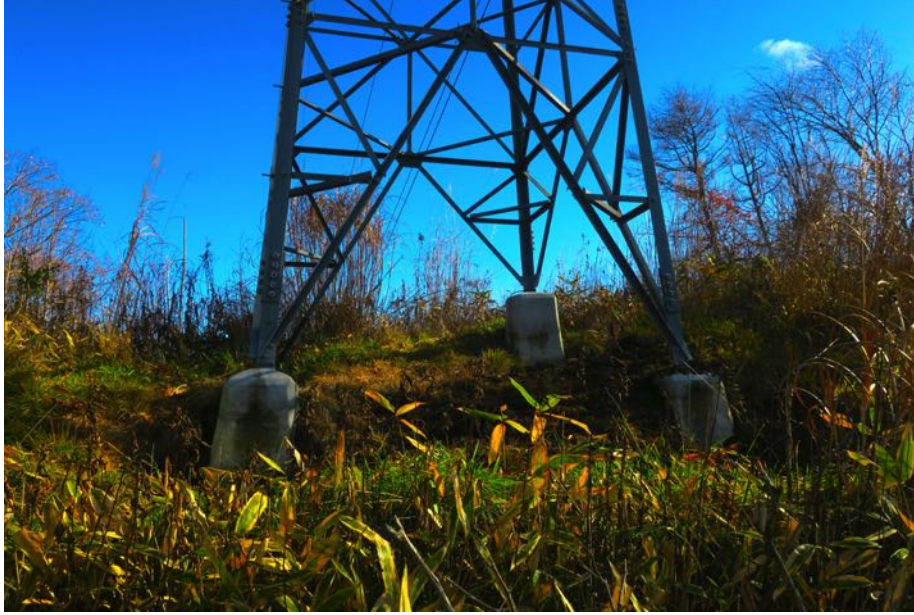
Figure 3-33. Head scarp beneath the tower in Figure 3-32 has exposed three of the four concrete piers
