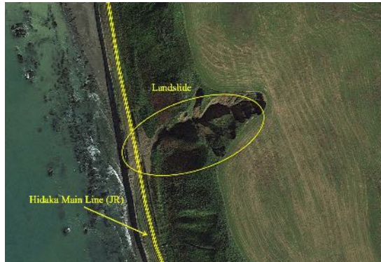
Figure 7-5. Landslide damaged the Track. (Source: Google Earth)
