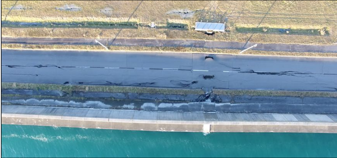
Figure 8-10. Aerial view of damage to the road and part of the seawall. (Source: Masataka Shiga)
