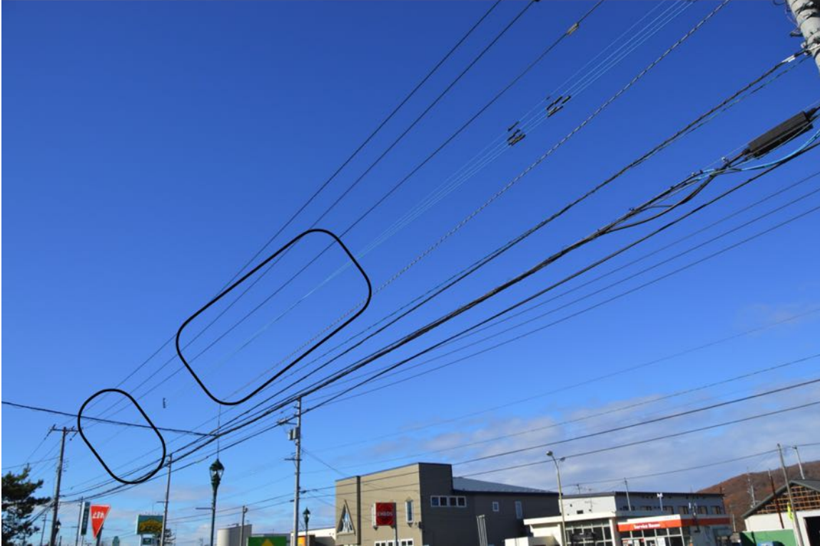
Figure 3-42. Wire Entanglement
