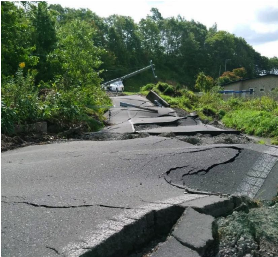
Figure 3-44. Toppled Distribution Pole due to PGDs along a Road (Atsuma-Cho) (Credit: HEPCO)
