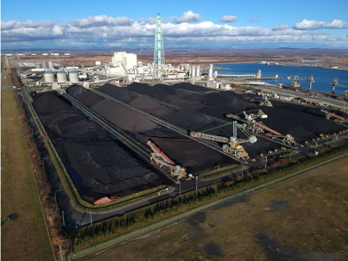
Figure 3-37. Tomatoh-Atsuma Power Plant (looking north)
