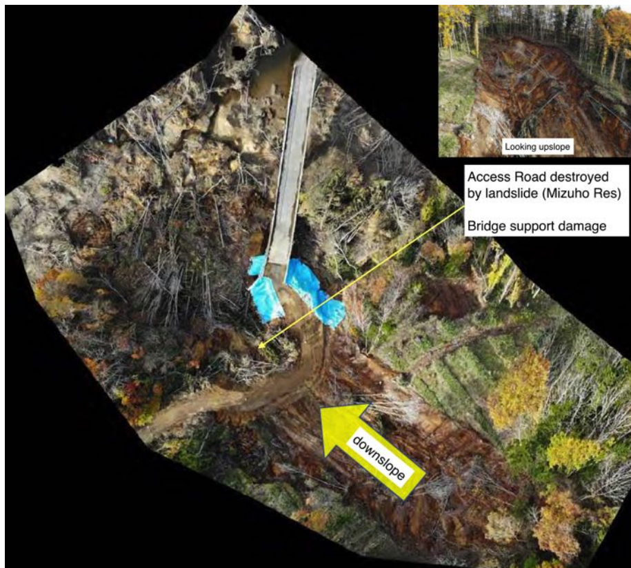
Figure 5-30. Access road destroyed by landslide at Mizuho Reservoir (photo: PG&E)
