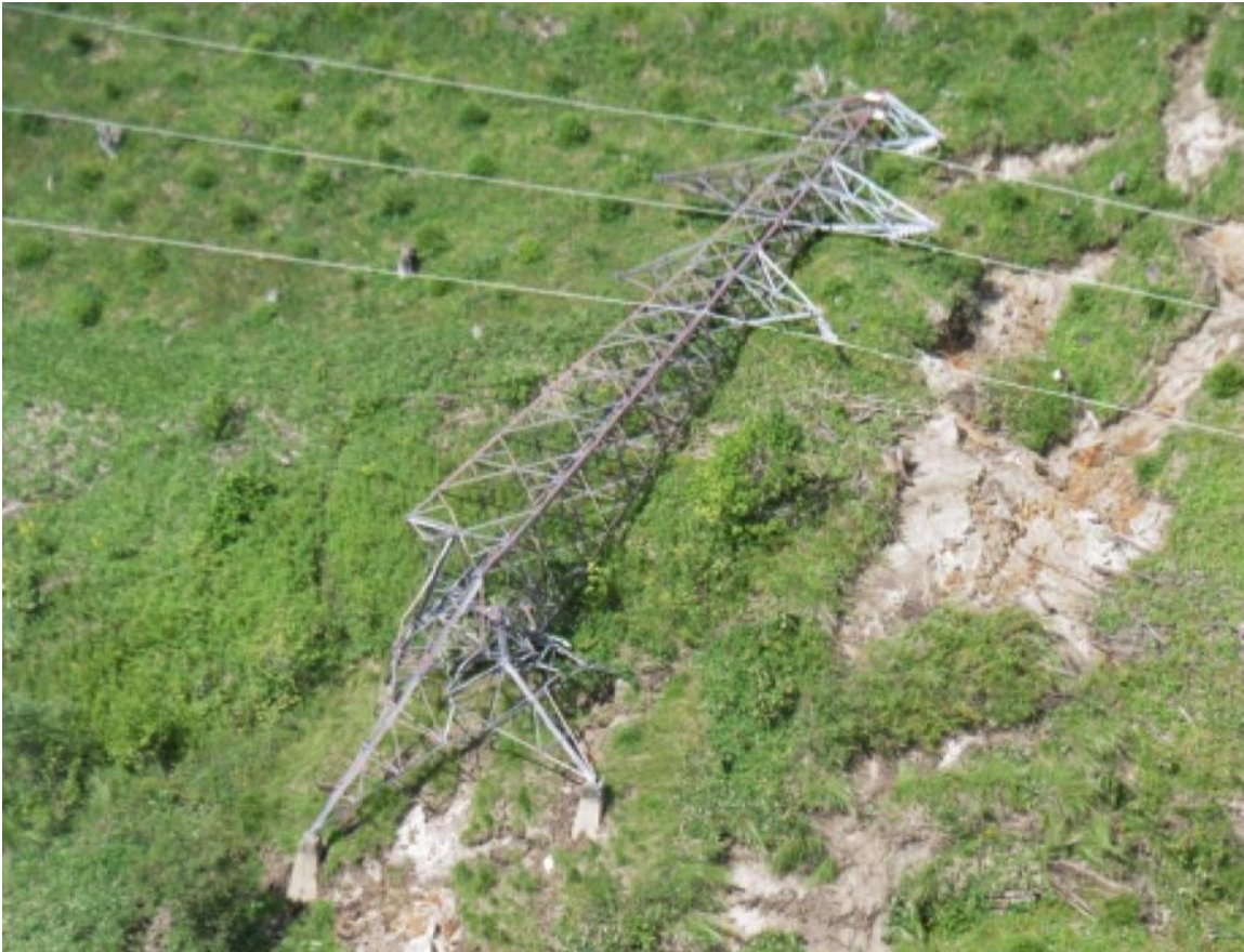
Figure 3-26. Collapsed 66 kV Tower 107 on Iwashimishi Line (credit: HEPCO)
