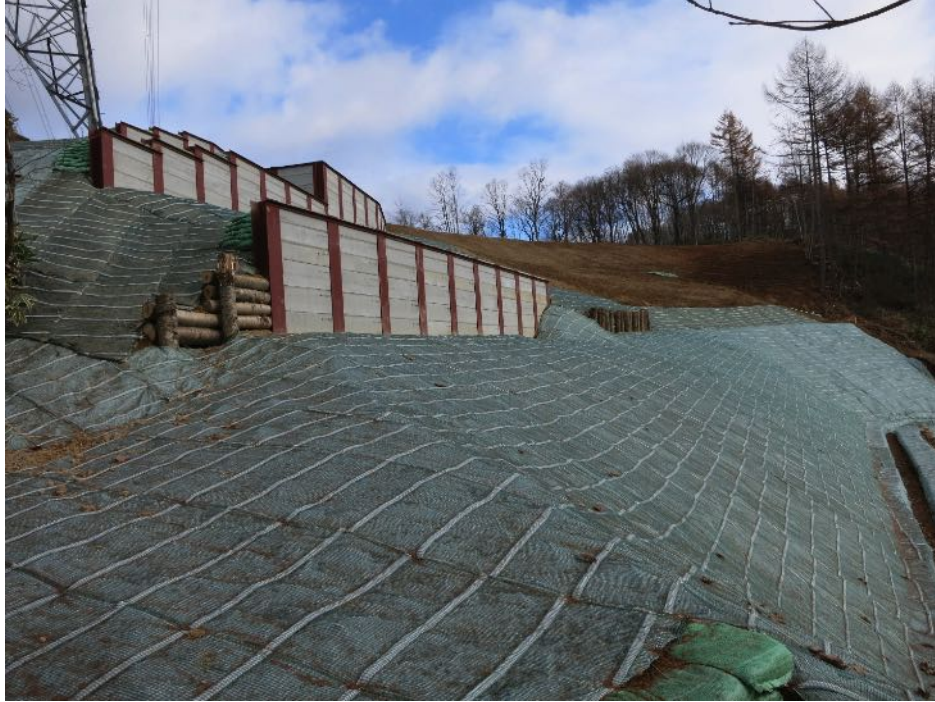
Figure 3-23. Benched Retaining Wall
